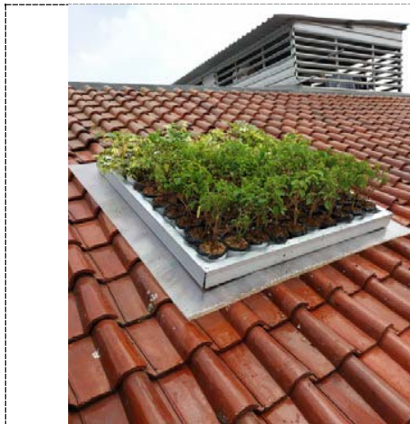
Figure 5. Roof garden model applied on sloping roof
