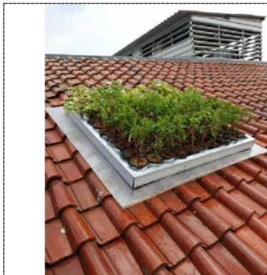
Figure 5. Roof garden model applied on sloping roof
