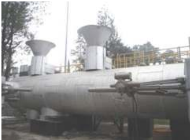
Gambar 5.11. : Contoh Steam Receiving Header
