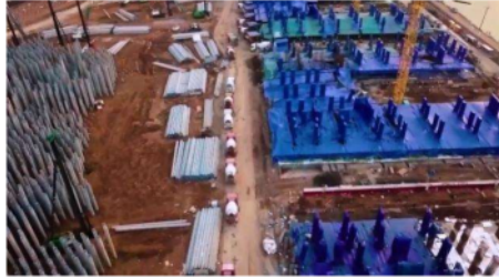
Fig.1 Tokyo Apartment Project using GGBFS
