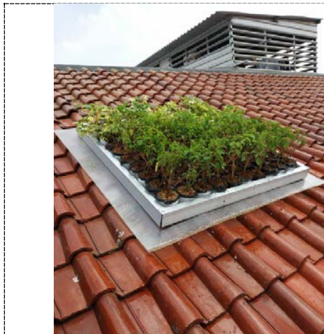
Figure 5. Roof garden model applied on sloping roof
