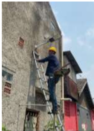
Gambar 6. Pemasangan Lampu LED tenaga surya
