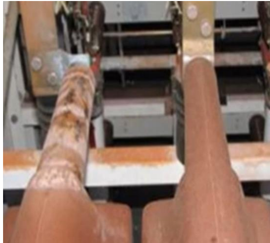
Figure 2 Corona tracks close to bus bars
