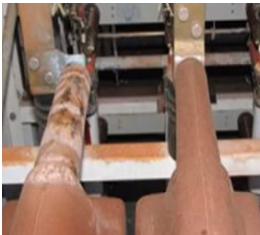
Fig. 2 Corona tracks close to bus bars
