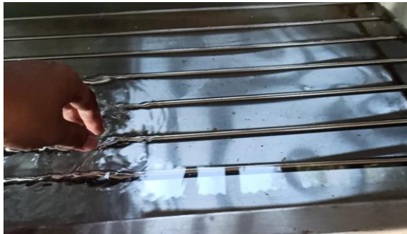
Gambar 16. Pipa Cooler Terendam Air
